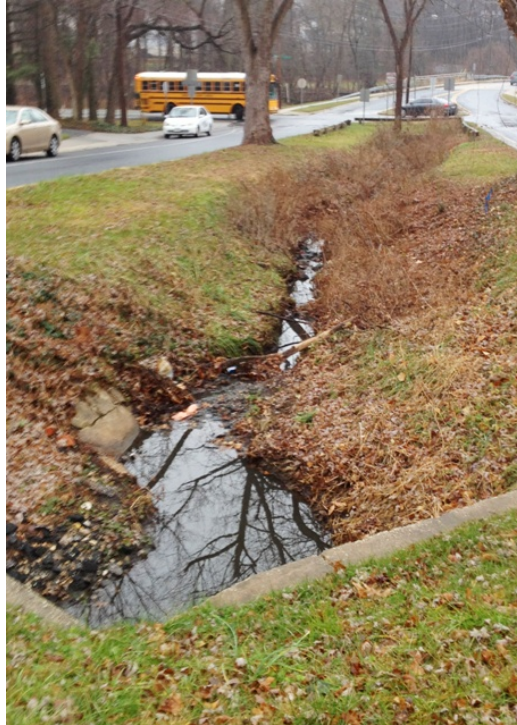
Figure 5.16: Regenerative Step-Pool Conveyance – Before and After
