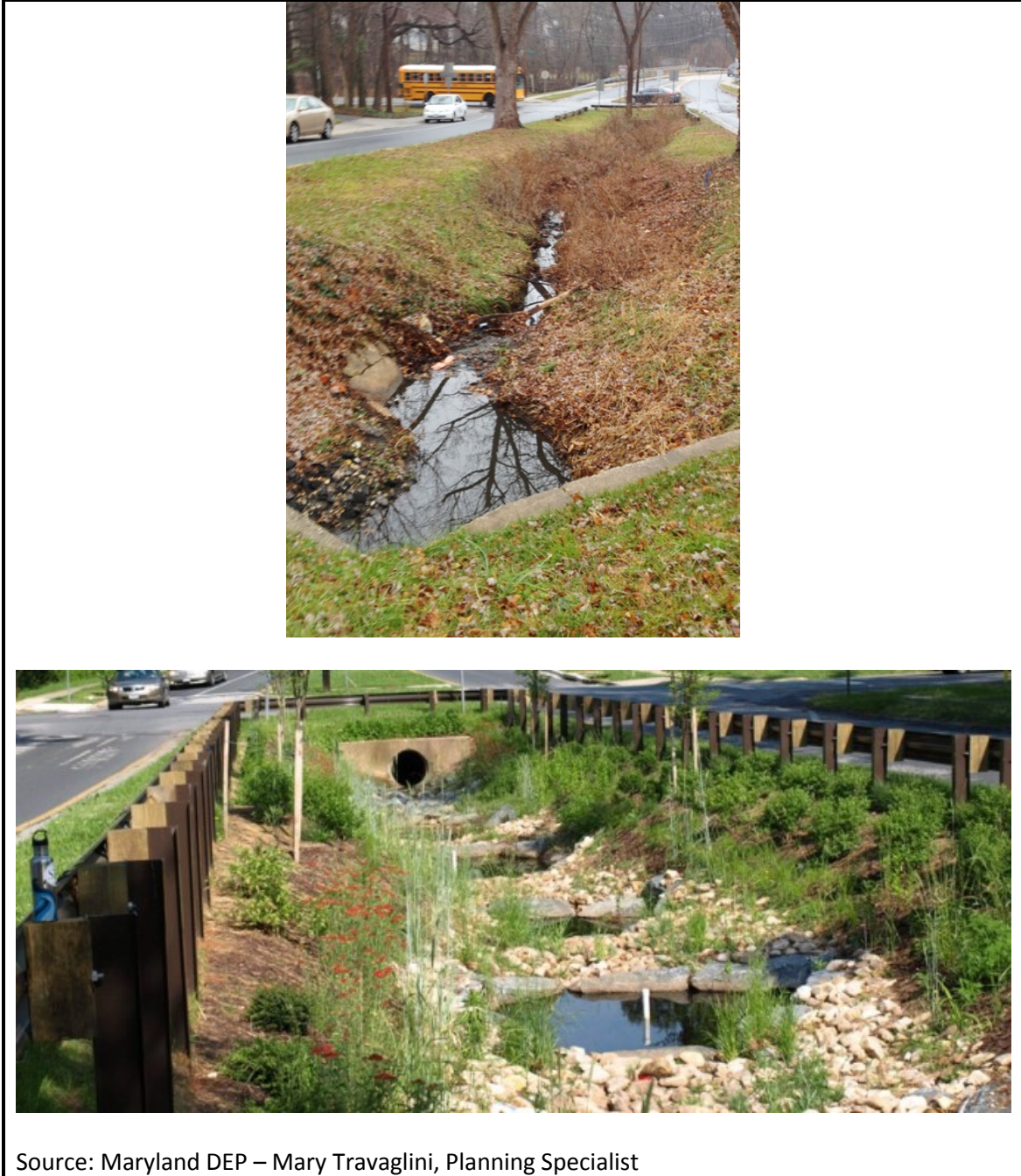
Figure 5.3: Regenerative Step-Pool Conveyance – Before and After
