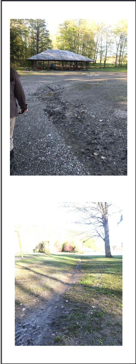
Figure 5.15: Parking Lot and Swale
