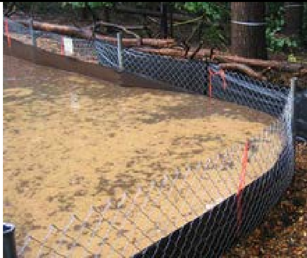
Figure 5.3: Example of Reinforced Silt Fence
