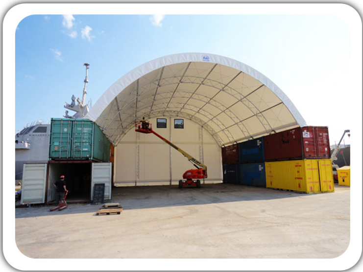
Figure 5.2: Example of Outdoor Storage Container
