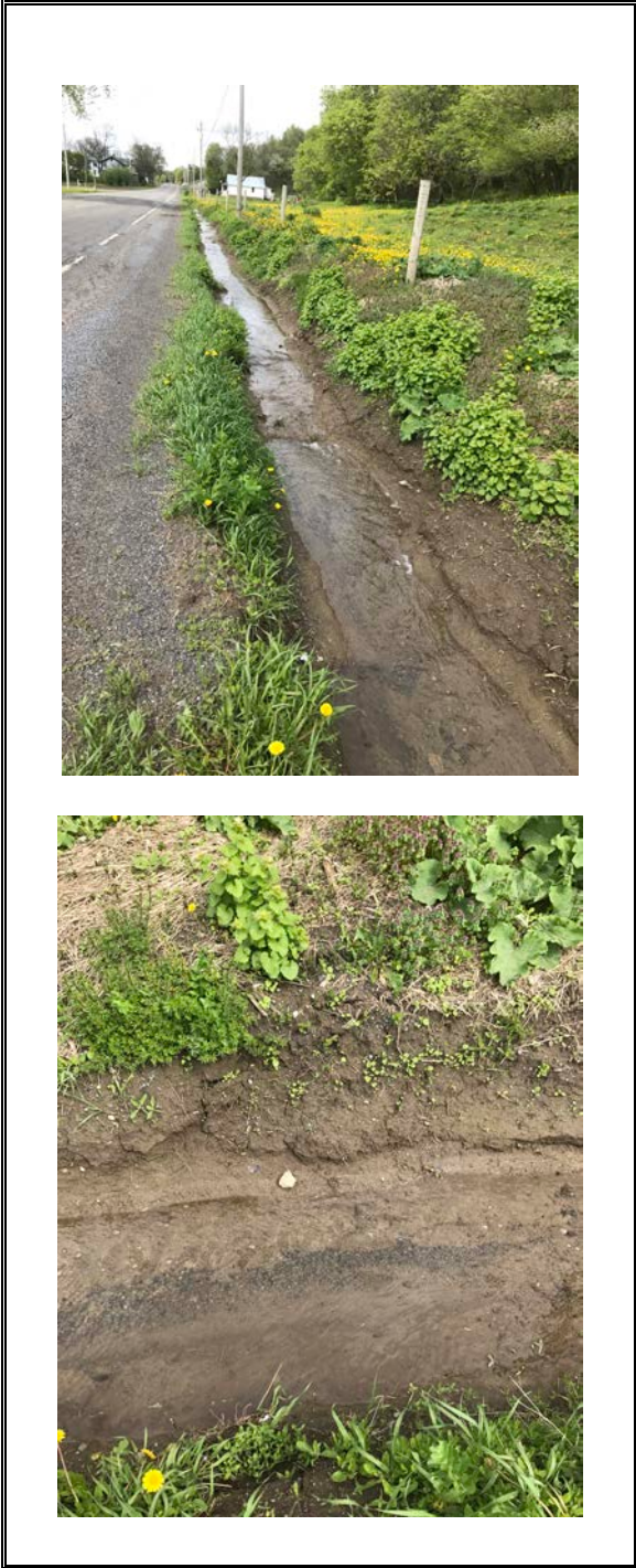
Figure 5.1: Route 11 Stormwater Ditch
